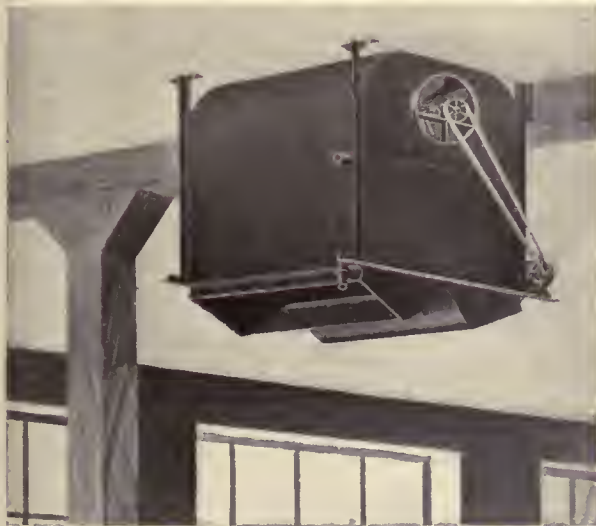
FIG. 11. TYPE OF UNIT HEATER SUSPENDED FROM CEILING
